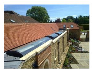
The project included the design, manufacture and installation of 3 No. Barrel Vaulted Rooflights along the length of the rear end of the listed building. Each rooflight was supplied in 3 glass panes to allow easy manual installation of the glass, however the glass to glass joints where produced in a frameless design thus maximising the natural daylight entering the space.
